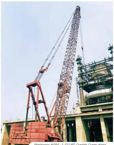
Manitowoc M250 -2 272 MT Crawler Crane doing structure erection job at site
